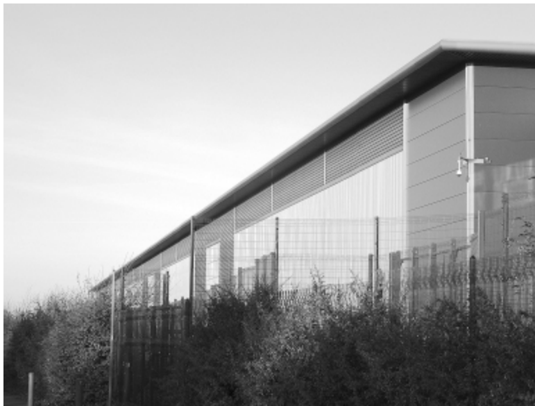
Photograph: James Bridle. NYSE Euronext Data Center, Basildon.
